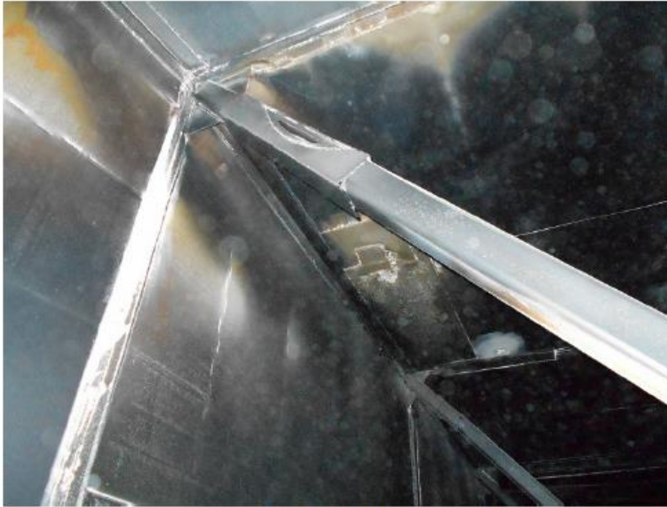
Internal truss erosion downstream of mixers (zoomed view at right)
