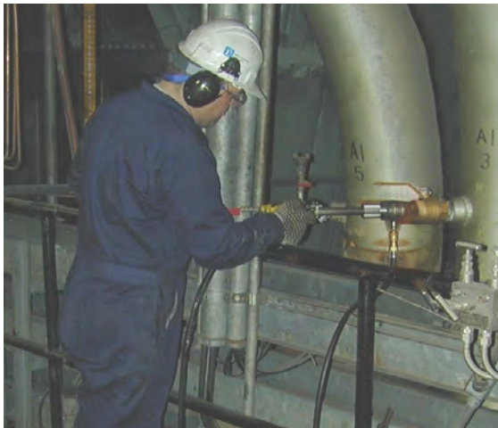
Particulate sampling in a coal piping system
