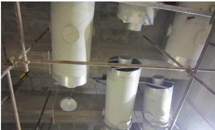
Isolated Phase Bus Duct Testing
